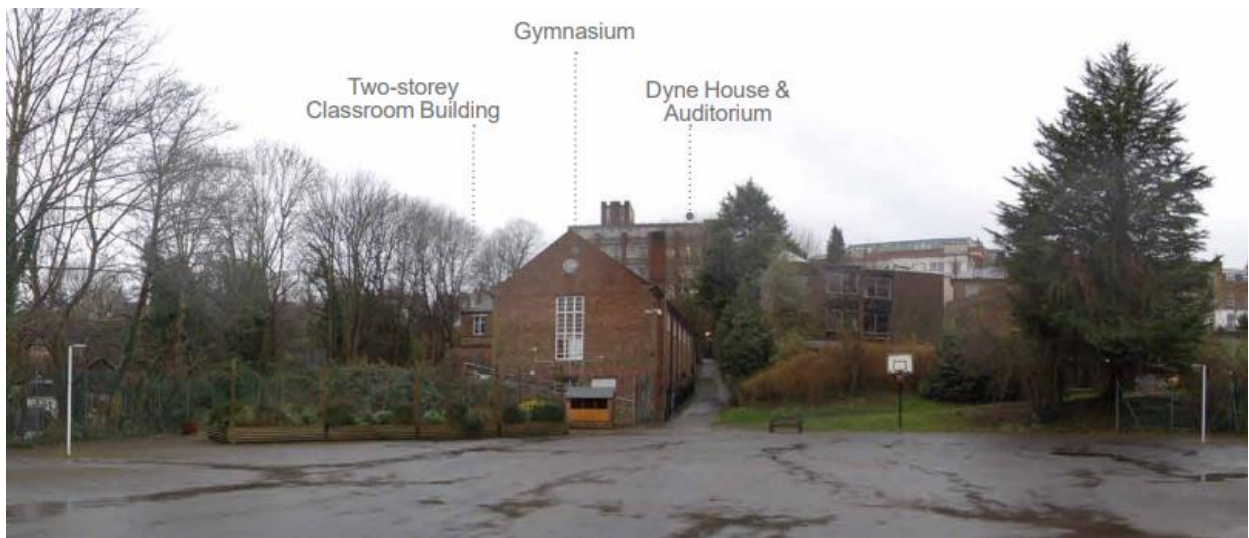
Photo of Rear Elevation
